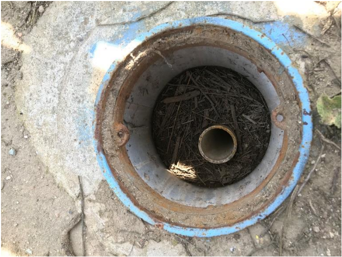
Figure 15. Monitoring well MW-6.
