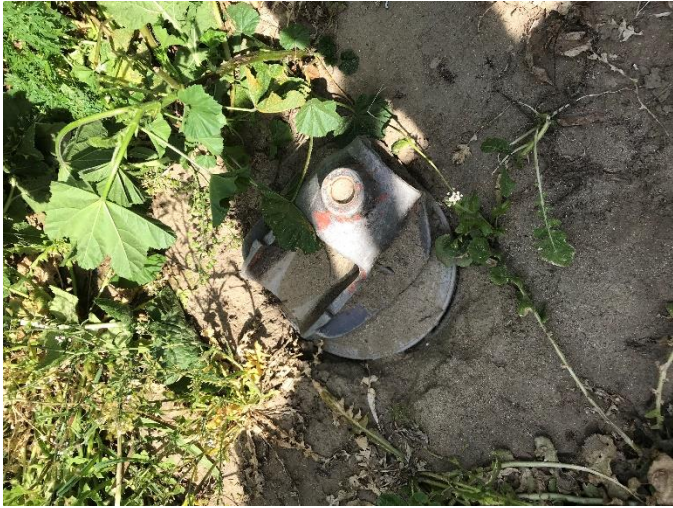
Figure 11. Monitoring well MW-4 overview.
