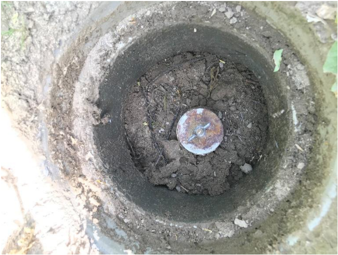
Figure 9. Monitoring well MW-4.
