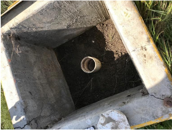
Figure 4. Monitoring well MW-2.
