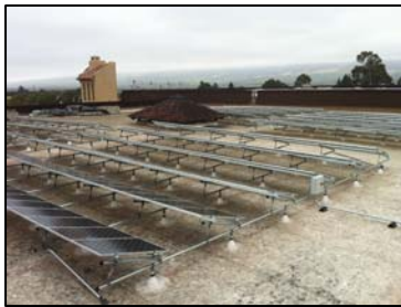
Solar project completed on the Constellation rooftop
