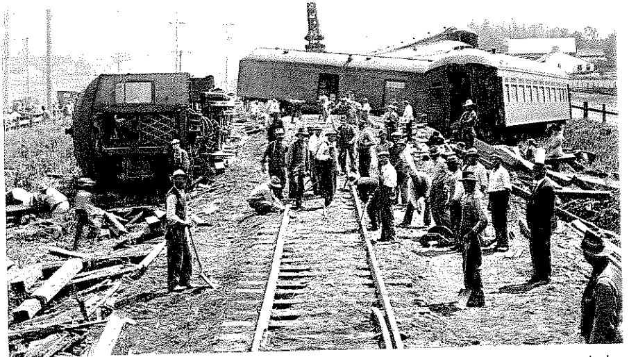
Gonzales' famous train wreck of 1915. A switch was left open and the above scene is what happened just at the north end of town.
