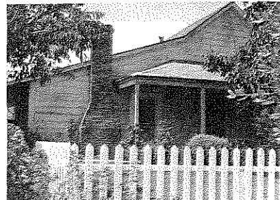
Albina Brusa home, oldest still standing. Don Schmidt photo.
