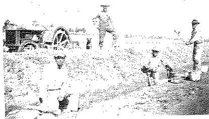
First concrete pipe laid in the Gonzales area. L. to R., Manuel Villa, Mr. Ferrasci, Lauro Pinon (father of Maria Marquez, Jane Pedroza and Alex Pinon), Alex Pinon. Pipe was all hand made by Pinon in Gonzales. Photo in 1927.
