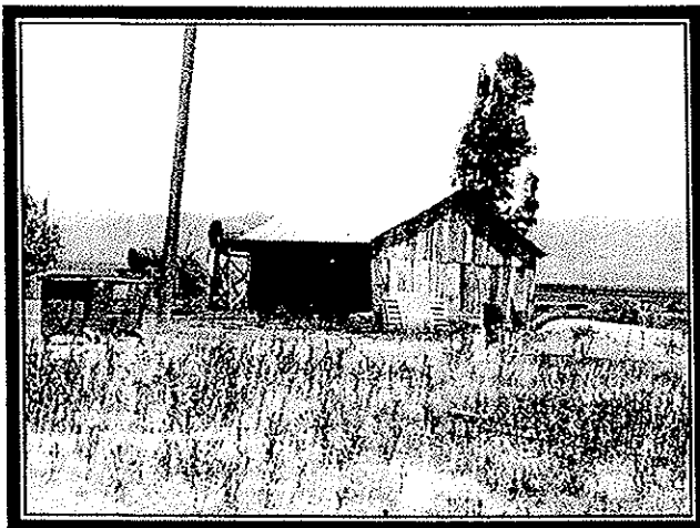
Equipment shed, southwest corner. 2000 photo.
